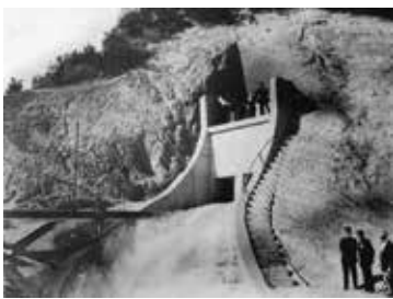
(1913) Opening Water Gates
